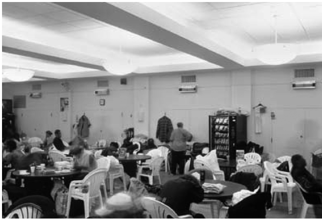
Fig. 7 Upper-Air UVC Treating Congregate Setting (TUSS Project, St. Vincent's Hospital, New York City)
